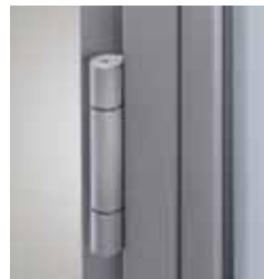
three-wing hinge h.90 | d.15 mm
