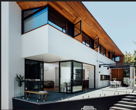
Architect: Pleysier Perkins | Builder: Wade Builders
